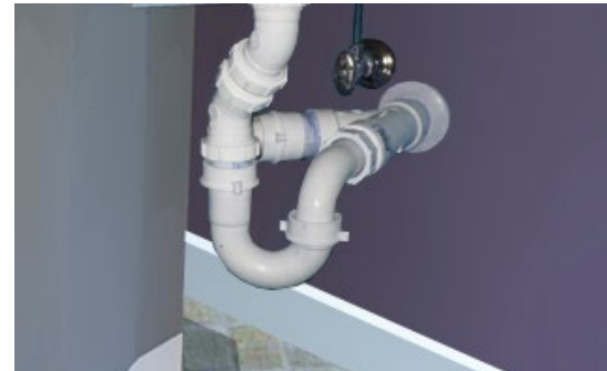
Seal gaps around pipes in interior and exterior walls.
