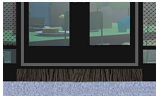
Install door sweeps on exterior doors.
